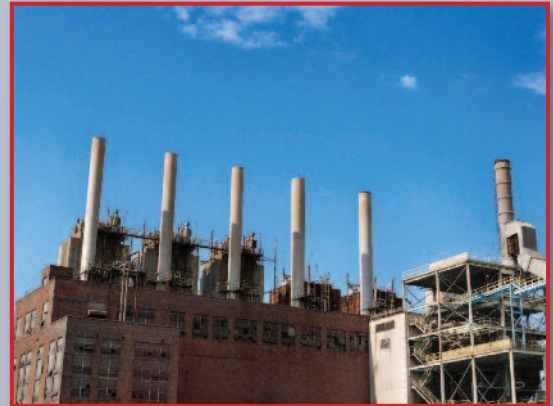
Industrial site inspection
